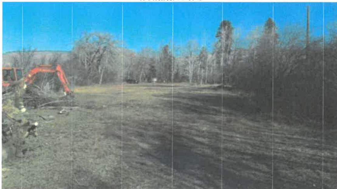
Below: Pasture area looking north just east of wooded area containing wetland A & B
